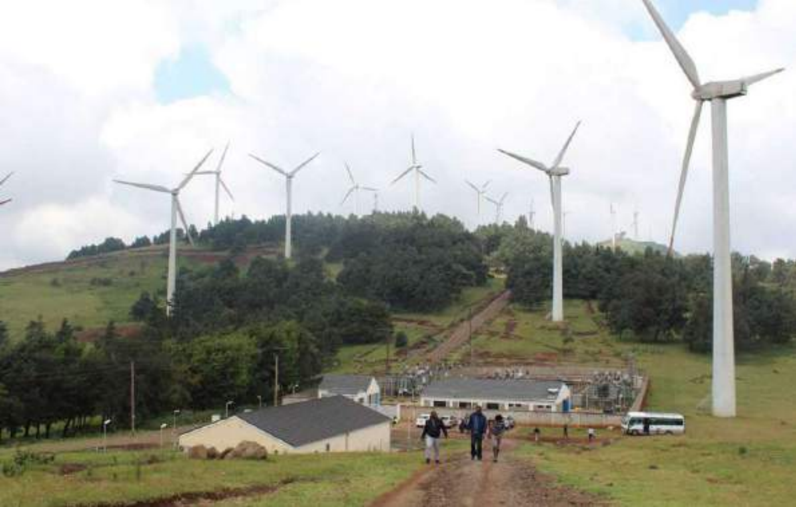
KenGen wind turbines and an electricity tower in Ngong Hills, Kajiado County. Kenya is lauded for achieving over fifty per cent electricity access rate (Photo Credit: The Standard)
